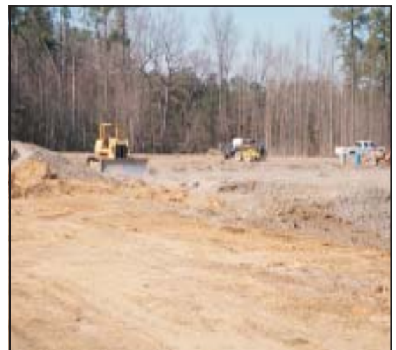
Site grading begins.
