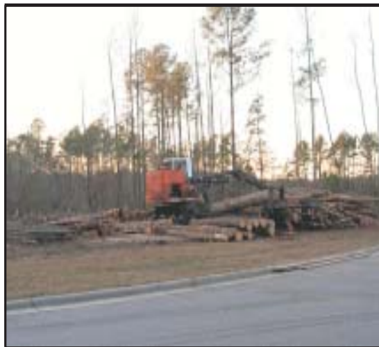
Site is cleared of excess trees.
